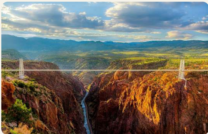
Bridge: the deck spans the gorge high above the Arkansas River.
